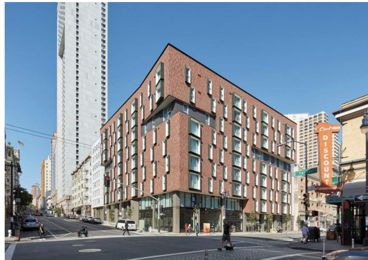
AFFORDABLE-HOUSING (THE EDDY, SAN FRANCISCO)
